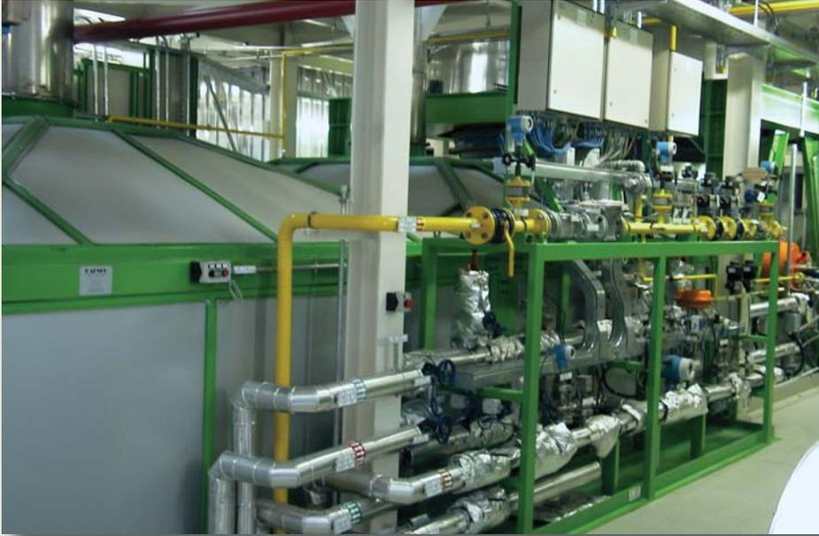
Rotary kiln plant with burner/Rack
