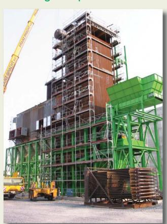
lates, plans and produces complete steam boilers of 5 – 150 tons with a pressure of 10 -110 bar and a temperature of up to 450°C.
